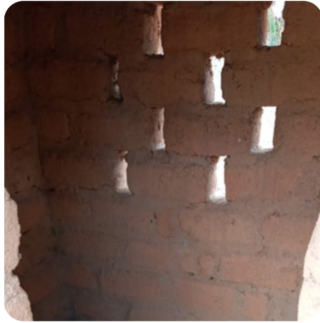
Vents in the wall
