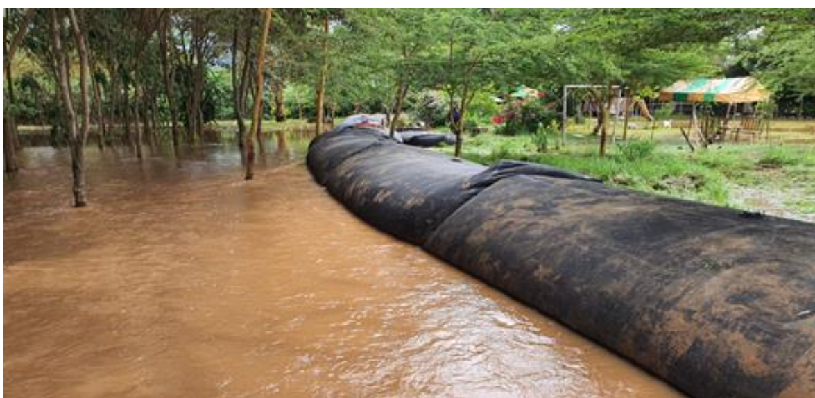
Using slamdams to protect the local pastoralists from flooding.
